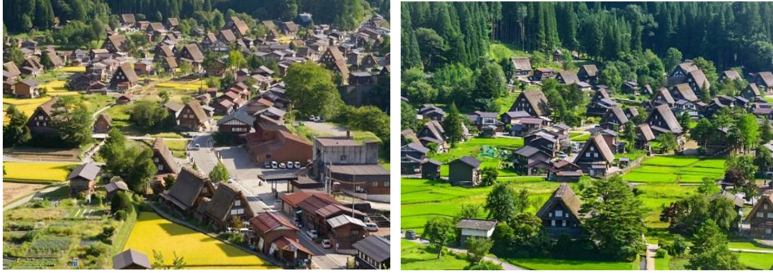
Şekil 3. Shirakawa-gō ve Gokayama (Gokayama and Shirakawa; Shirakawa-go & Gokayama, 2025) Hahoe ve Yangdong – Güney Kore (Şekil 4)
