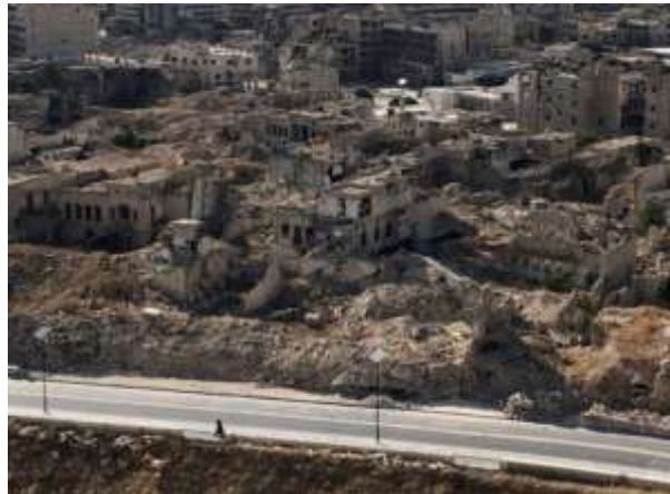
Figure 3. War destruction near the Aleppo Citadel. (Bandarin, 2016, )
