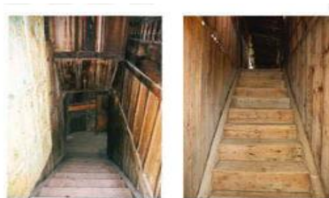
Figure 13: Stairs construction In the Village(Sağiroğlu, 2017).
